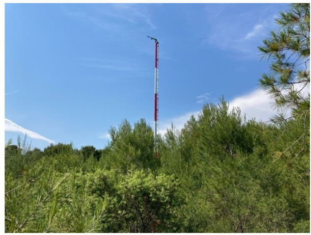
Figure 3. Left: Tower at Masia Traver site, painted in green to achieve landscape integration. Right: Tower at Cañada Sur site, painted in white and red strips in accordance to airport regulations.
