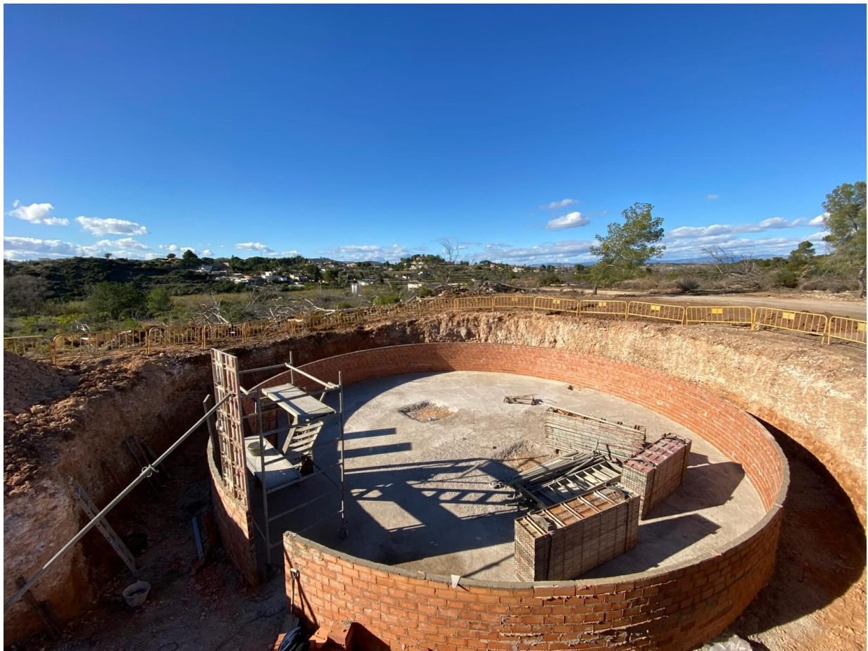
Figure 4. A GUARDIAN recycled water storage tank under construction.
